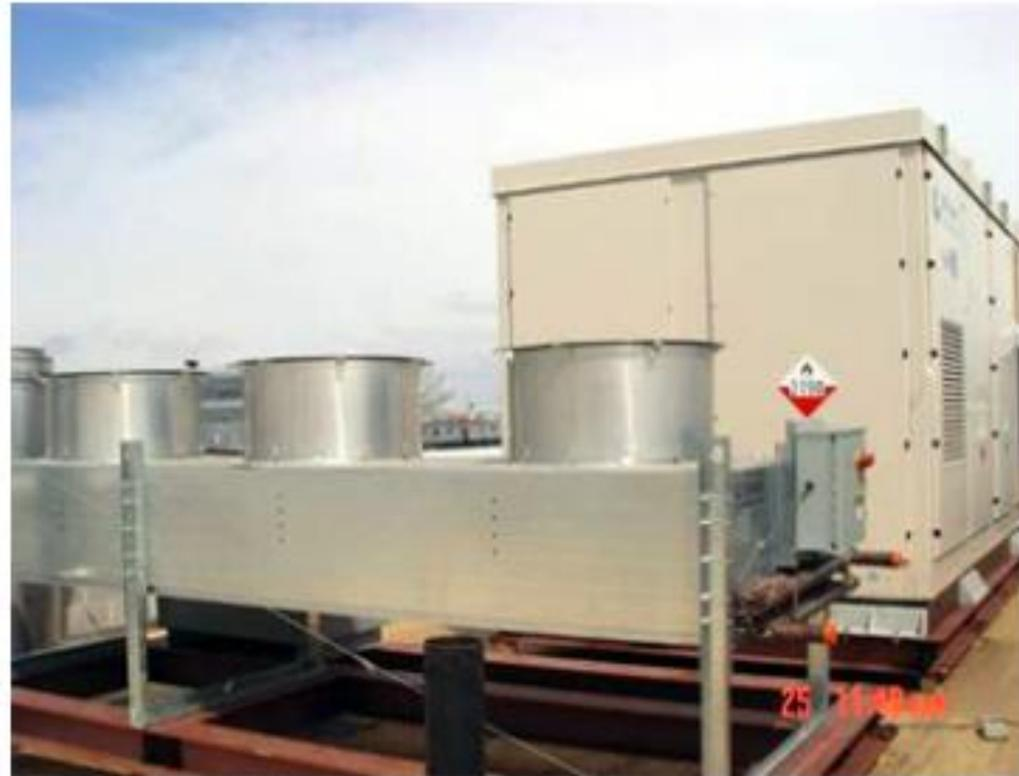
This fuel cell (background) converts hydrogen and oxygen into electricity and heat to save energy.
