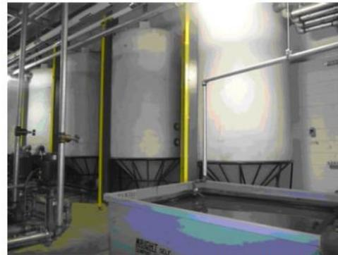
After the wash, the now "gray" rainwater goes into this blue bin. The white tanks filter the water.
